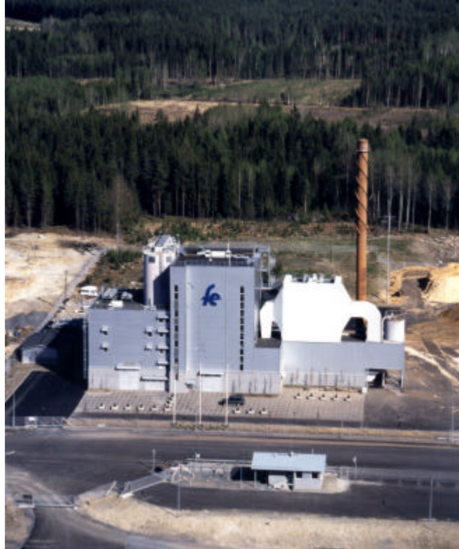
Figure 16. Forssa CHP plant using wood chips and wood residues /2/.
