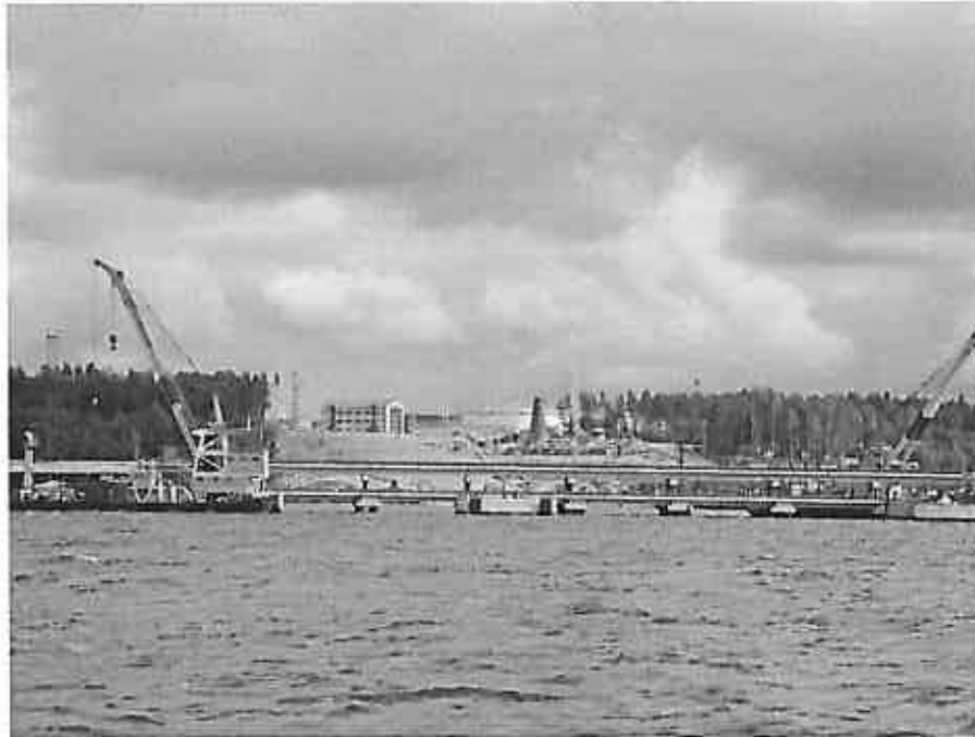
Figure 2. Primorsk oil terminal under construction in autumn 2001.
