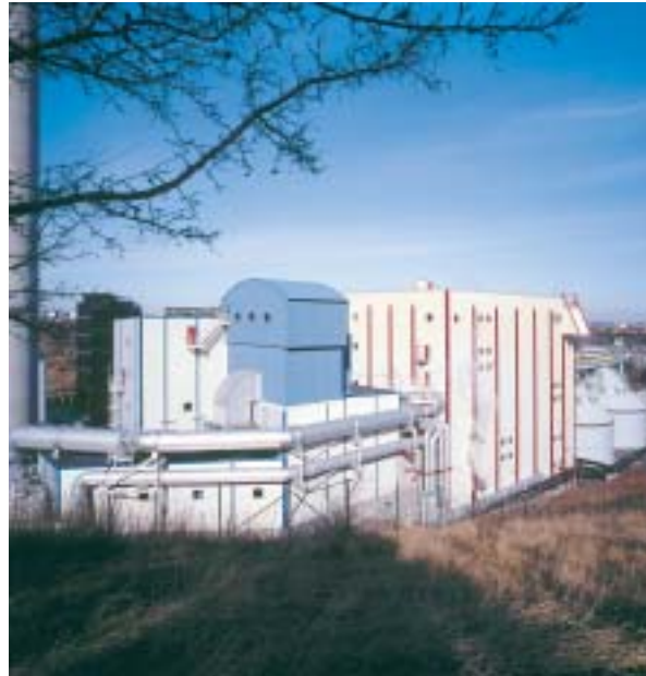
A circulating fluidised bed boiler (91.2 MW) of Birka Energi, an energy utility in Högdalen, Sweden, burns recovered fuels with forest residues, sawdust, bark and wood pellets. Foster Wheeler.
