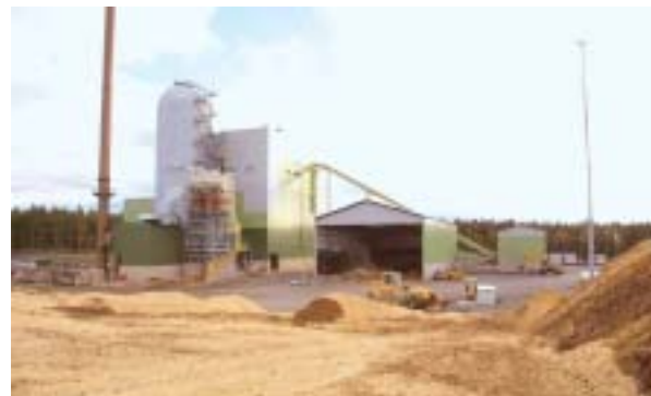
The main fuels of the Kokkola power plant in Finland are wood-derived fuels and peat, which can be stored in the fuel yard. In the basic planning, special attention was paid to a flexible selection of fuels on an extensive range of partial loading without the risk of corrosion. The Kokkola power plant is producing 20 MW e of electricity and the output of the BFB-boiler is 70 MW th . Pohjolan Voima Oy.
