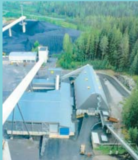
Fuel receiving stations and coal yard. Roxon.
