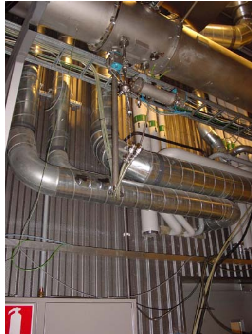
Figure 13. Full CVS tunnel for heavy-duty vehicles.
