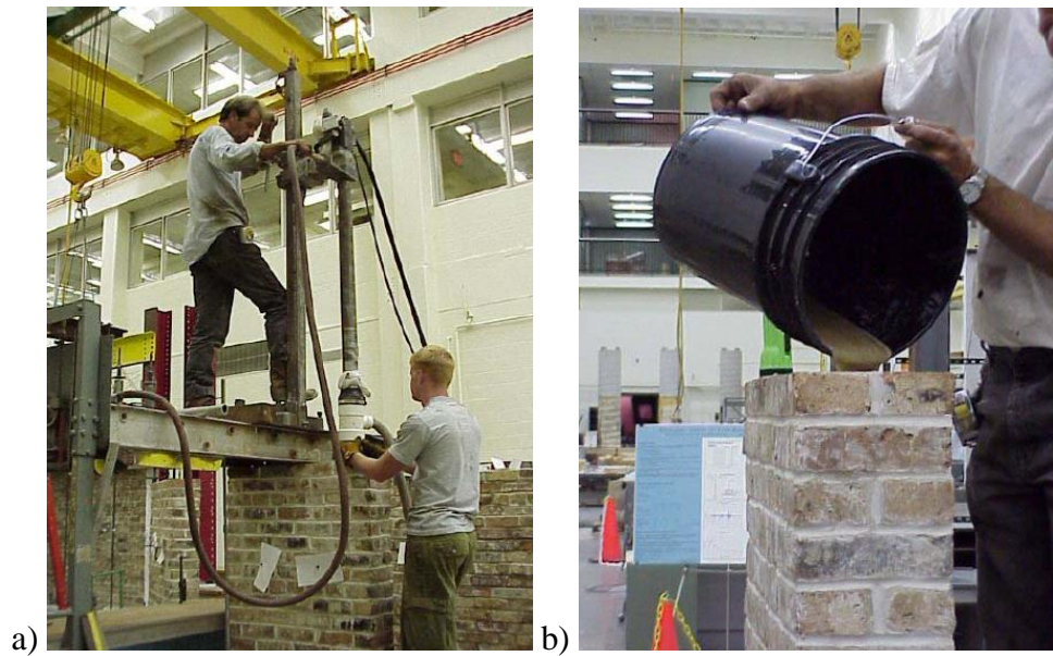
Figure 10. (a) Hole drilling and (b) grouting for centre-core rehabilitation in laboratory [6]
