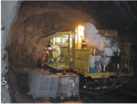
GroutAid at work in the Oslo Metro extension project
