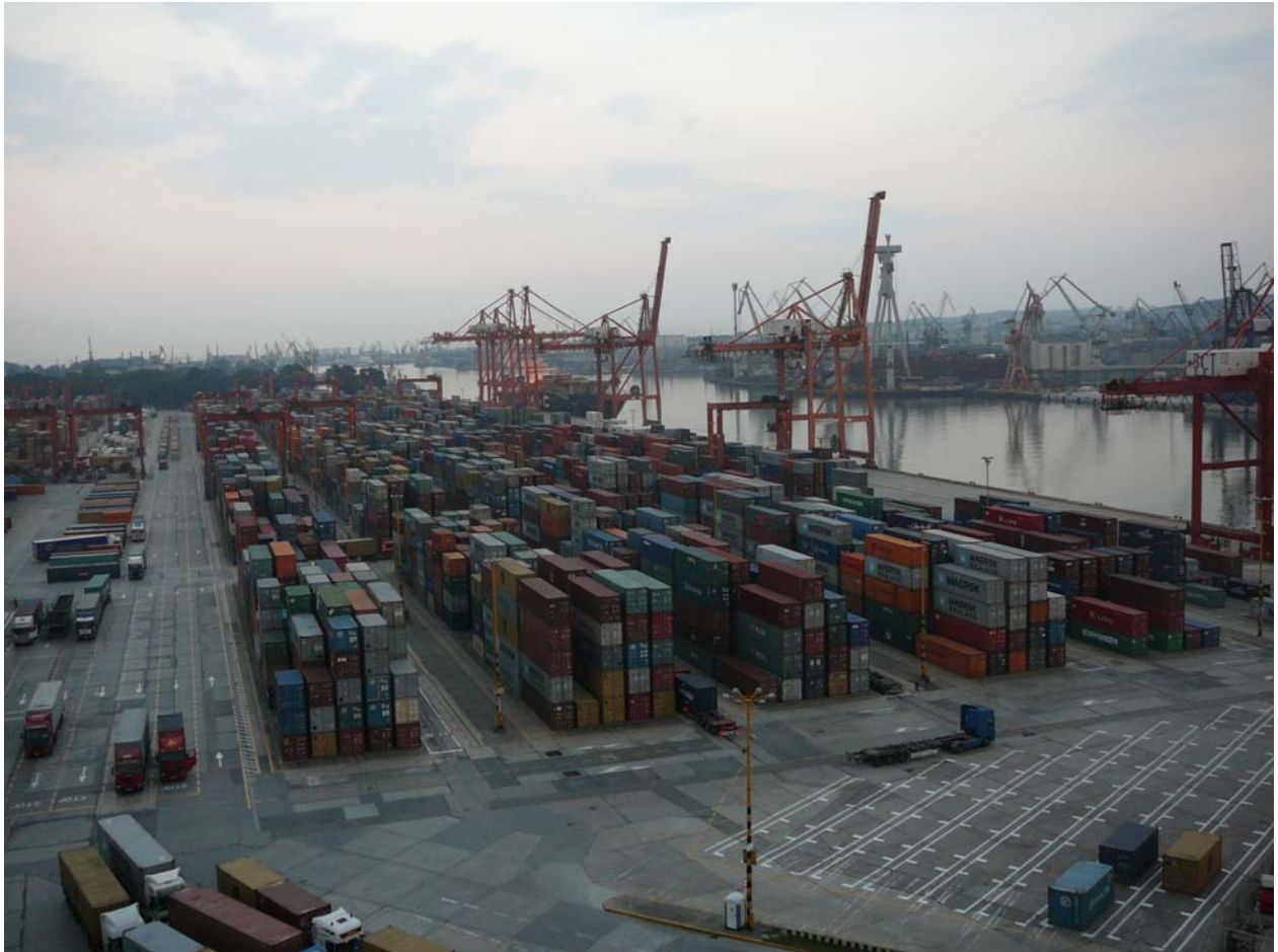
Figure 20. Port of Gdynia intermodal terminal.
