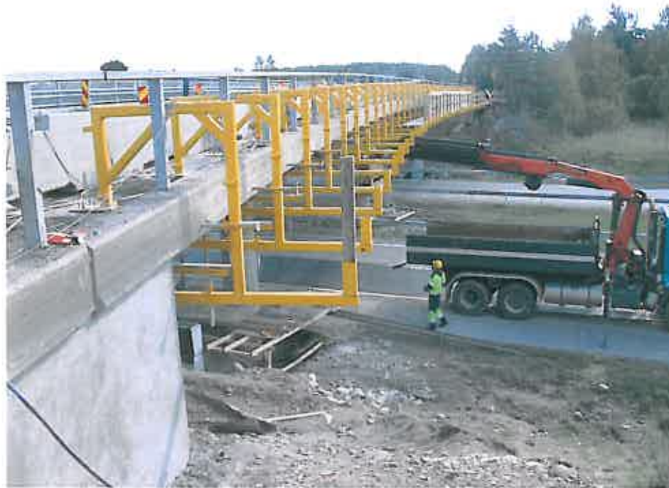
Figure 4.1. Boxby concrete bridge in Sipoo during rehabilitation.
