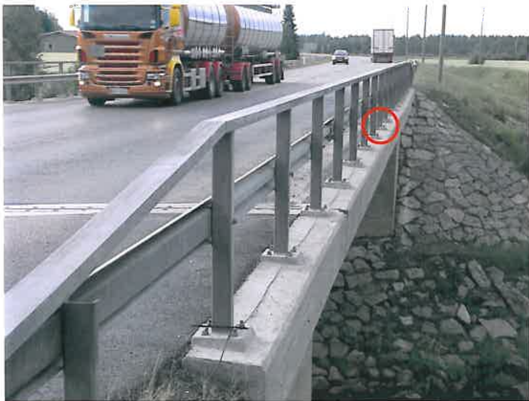
Figure 6.3.3. Accelerometers location (circled).
