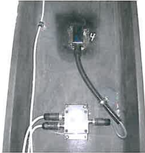
Figure 3.1.2. Strain gage installation.
