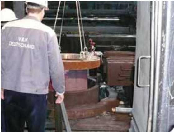
Removal of the centralising device
