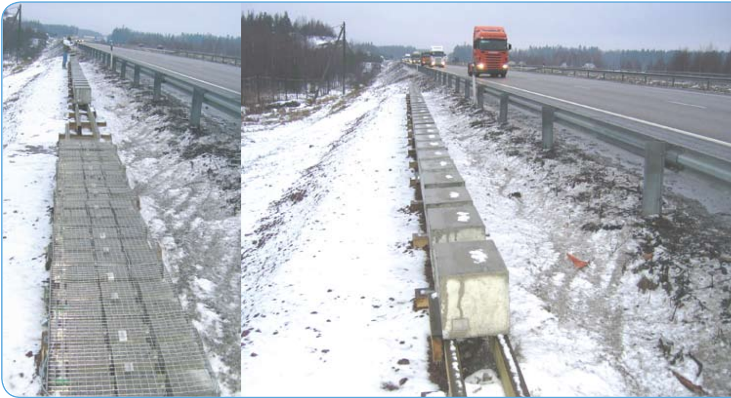
Figure 1. Highway 7 in Finland, frost-salt and chloride penetration samples.
