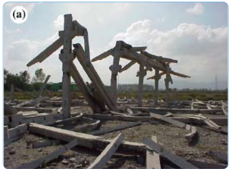
Figure 1. Collapse of unfinished precast structure in the August 17, 1999, Kocaeli (Turkey) earthquake [1].
