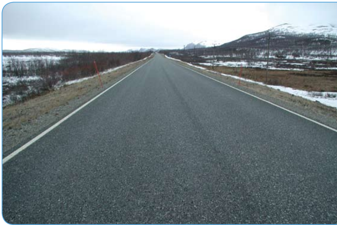
Figure 1. Example of use of moraine from earlier trial test of low-volume road.
