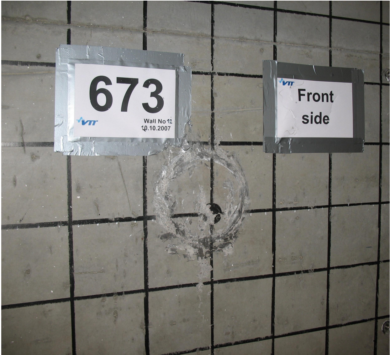
Figure 91. Front surface of the wall in Test 673.
