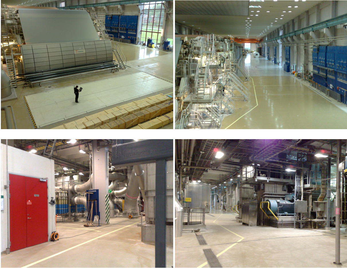
Figure 46. Pictures from the pilot area on the operation floor.
