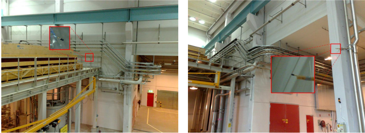
Figure 50. The small helix antennas of the pseudolites number 1 (left) and number 5 (right).
