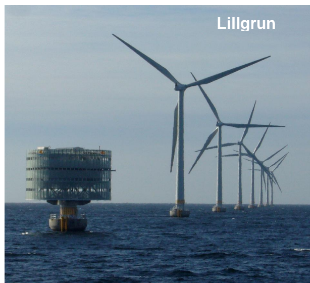
Figure 3. Example of an offshore wind farm from Sweden (Lillgrund 110 MW, 48 times 2.3 MW).
