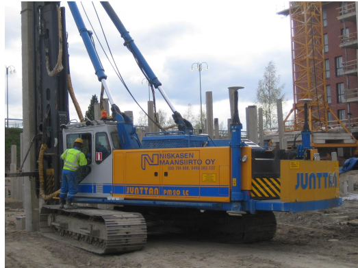
Figure 4. Junttan PM-20 piling rig.
