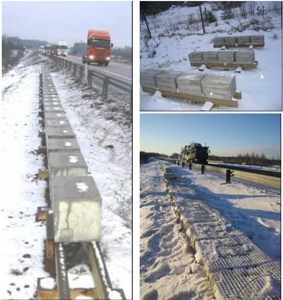
Figure 4. DuraInt field exposure at Highway 7 (HW 7 field, Kotka). Large specimens for chloride penetration are placed on wooden stands. Specimen for frost-salt testing are also on wooden stands, but in metal racks.
