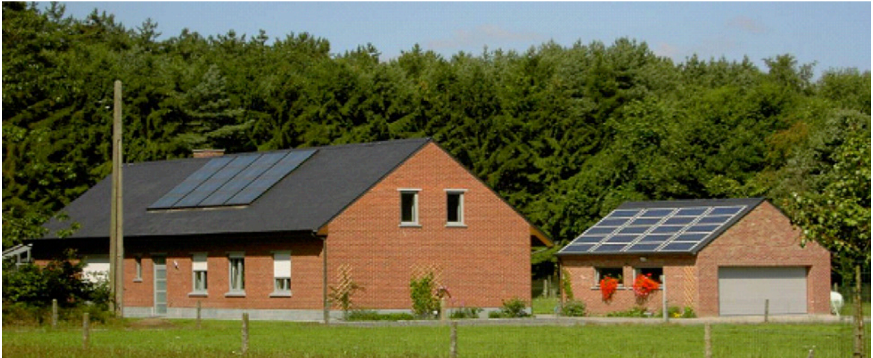
Retrofit of a century old country house into a low energy house, Herstelt, Belgium, architect: S. Corten [9]
