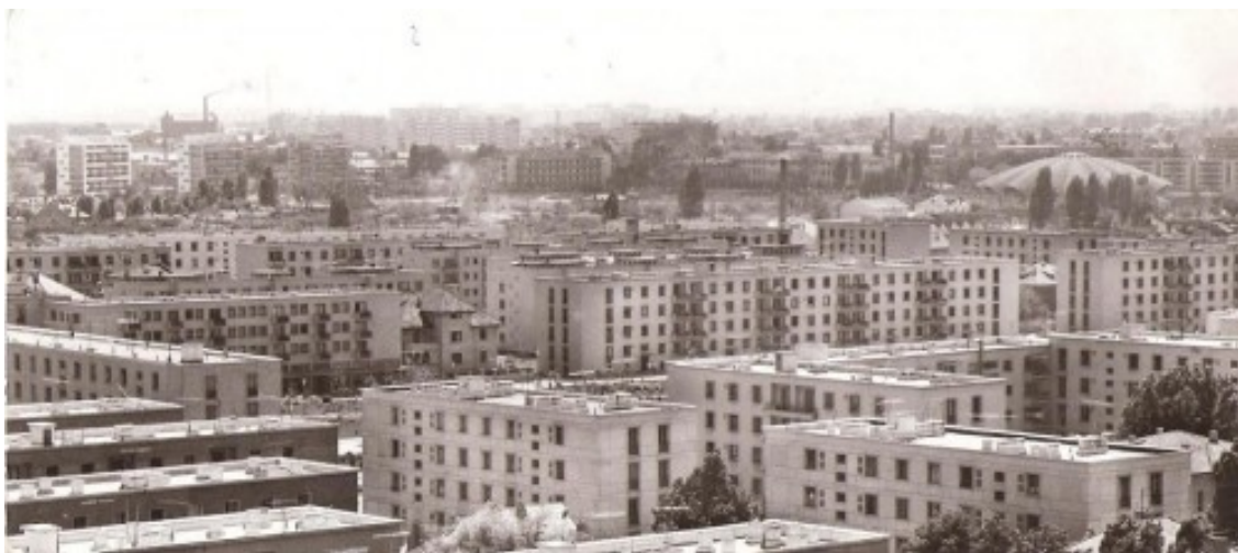
Figure 2. Typical apartment block area.
