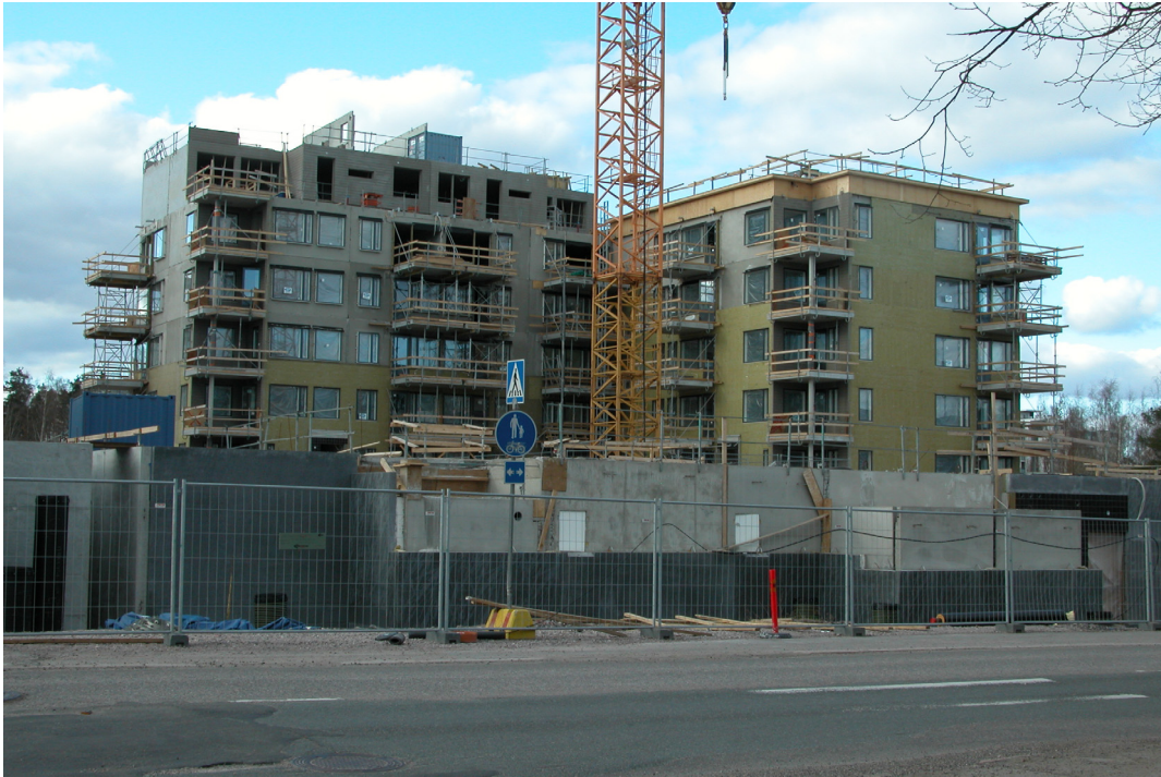
Figure 1. Ongoing construction using prefabricated concrete panels in Espoo, Finland (2010).
