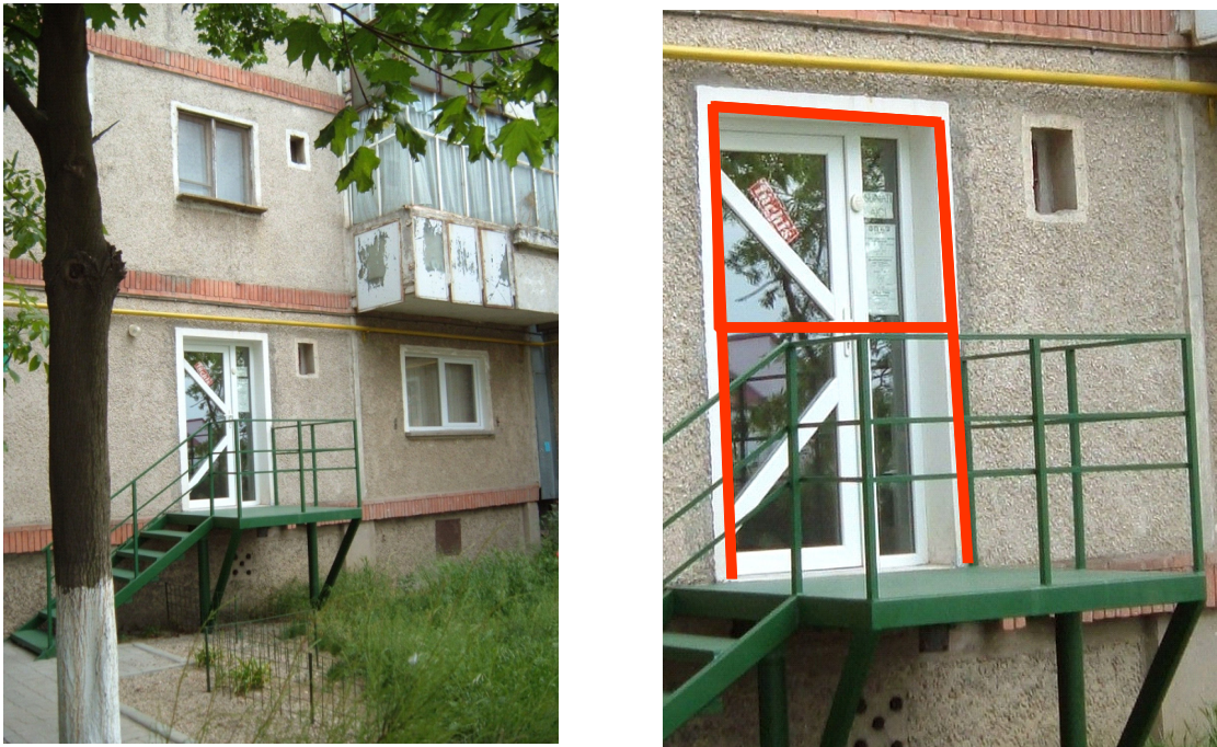
Figure 2. Typical example of structural remodelling by doorway cut-outs.
