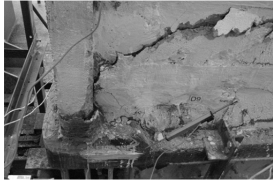
Figure 16. Diagonal crack reopening
