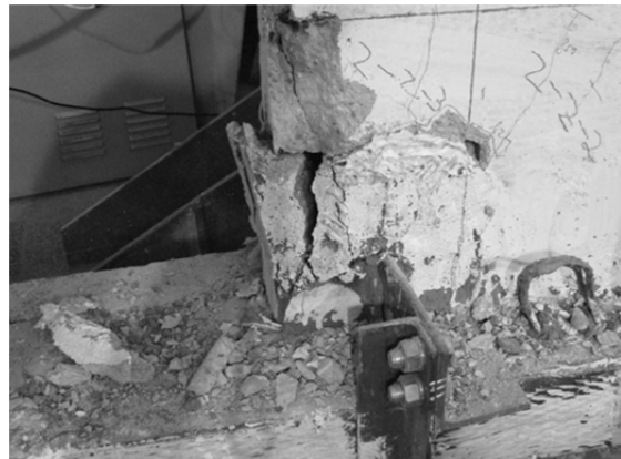
Figure 20. Cast in place mortar crush
