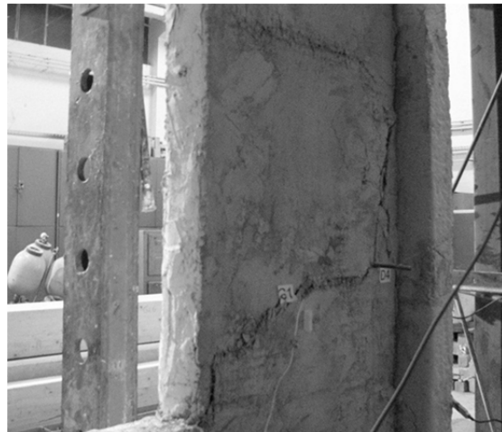
Figure 30. Rear view of the left pier [10]
