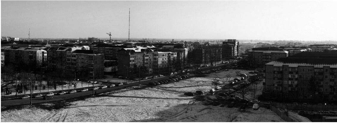
Figure 3. The Soarelui Neighborhood, Timisoara – where we can see clearly the effect of the first measure mentioned previously – almost all the apartment buildings in the area have attics instead of terraced roofs, which leads to an increased indoor comfort.
