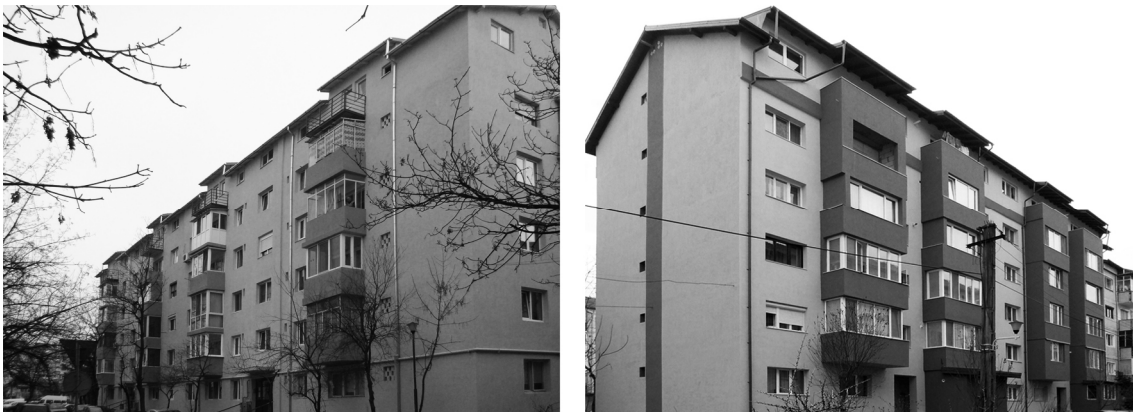
Figure 4. Timisoara – apartment buildings recently refurbished within the Dambovita Neighborhood and the Soarelui Neighborhood.
