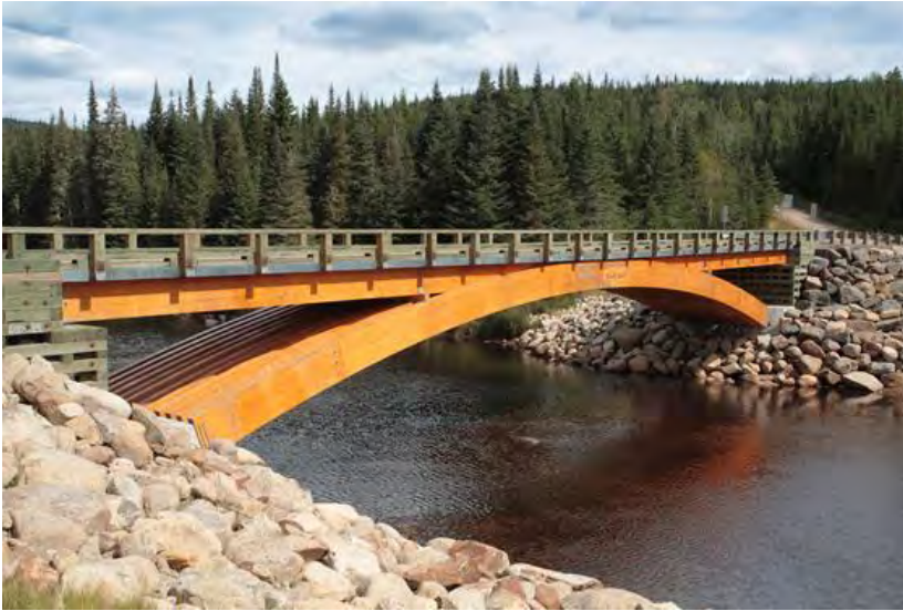
Figure 7. Wooden bridge in Montmorency River, Quebec, Canada (Wikipedia Creative Commons).
