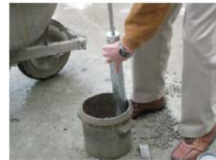
First lift compacted
