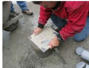
Striking off the surface
