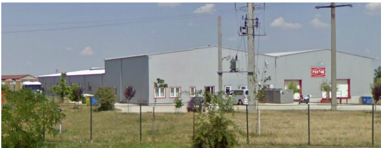
Figure 18. Industrial building in Arad (Romania).
