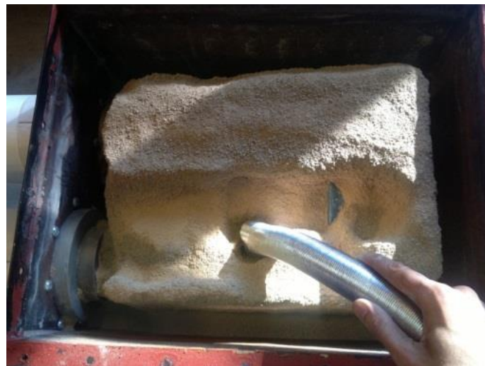
Figure 12 Removal of the granular insulation by vacuuming after the experiments. Note how the granules have bonded together forming a uniform insulation block.
