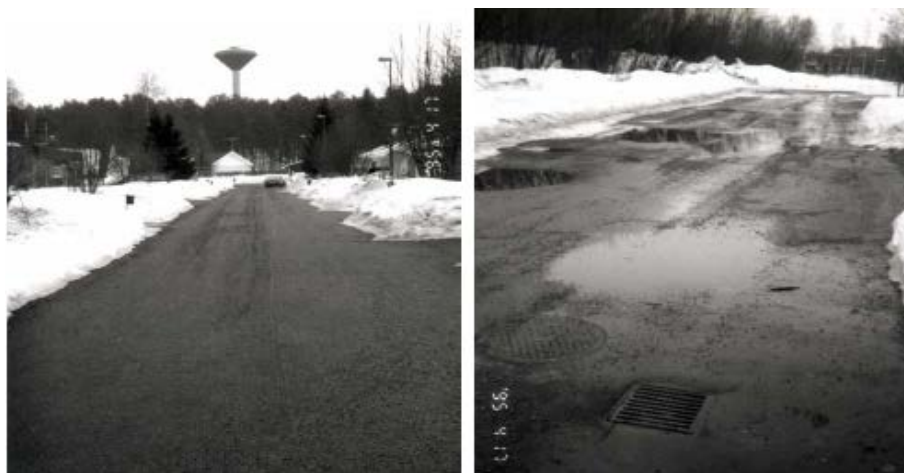
Figure 11. Comparison of porous pavement (left) and a nearby impermeable pavement (right) during the snowmelt period. [Hogland & Wahlman 1990, Westerlund 2007]
