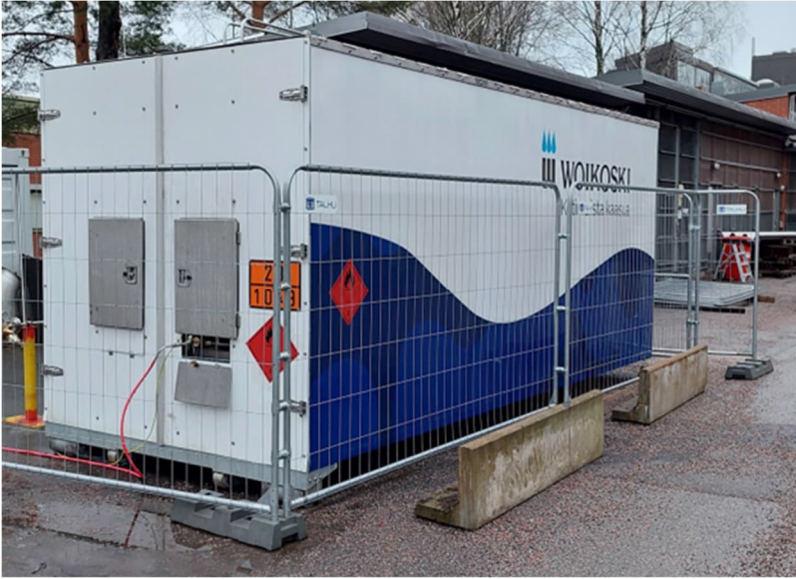
Figure 27: VTT Hydrogen storage at the outside of the test facility.
