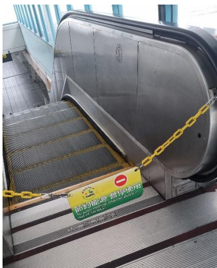
Figure 5 An escalator at a metro station in Taipei with a sign of being shutdown to conserve energy. Image: Arho Suominen
