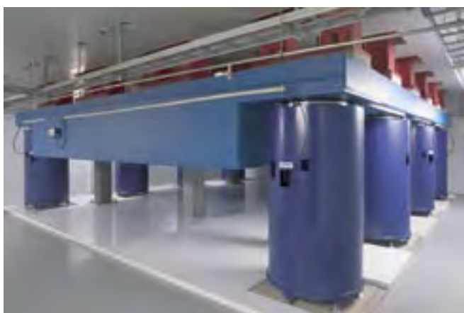
Figure 1. 140-ton slab on top of which are the measurement tables of two mass laboratories. For somewhat more modest vibration isolation some laboratories have been based on gravel-isolation carpet-concrete slab-structures. The third main solution is concrete plinths mounted on solid rock.
