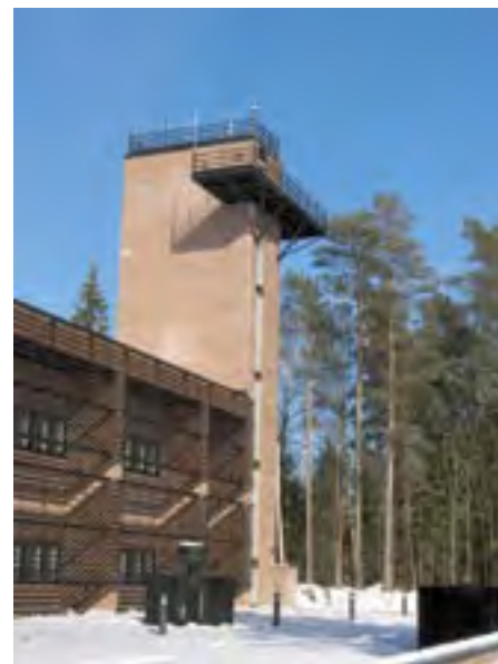
Figure E2. The antenna and receiver for the GPS common view measurements are located in the "clock tower" of the new MIKES building.
