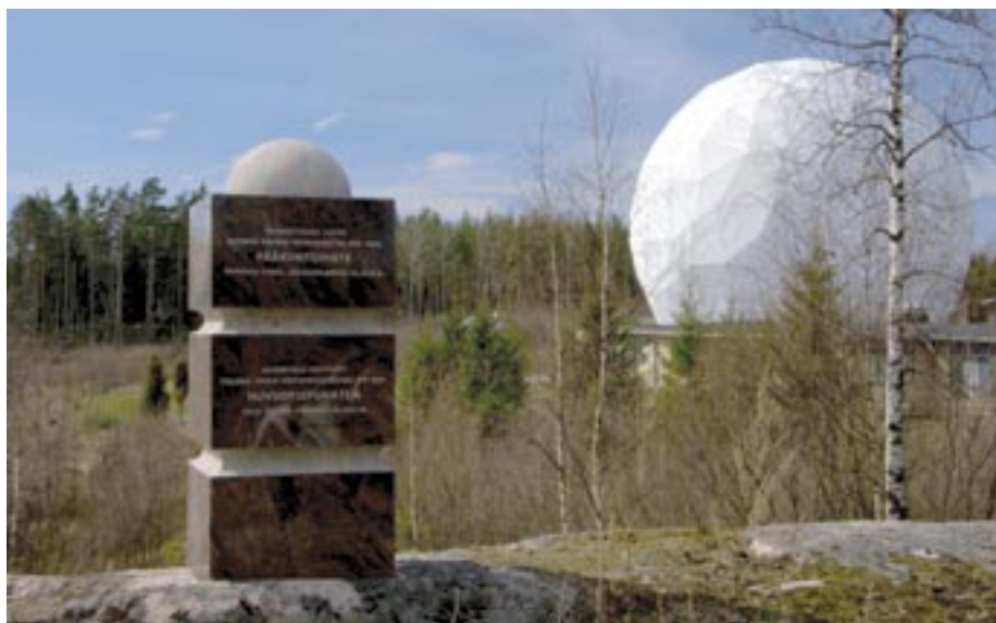
Figure L4. The main benchmark of the new Finnish height system N2000 is buried under a granite monument. The radome of the VLBI telescope is in the background.
