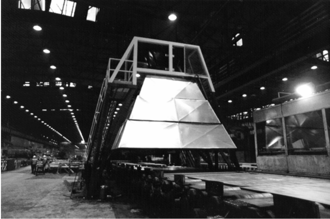
Figure 14. Installation of the measurement unit in the plate mill.
