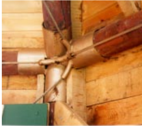
Figure 5.31. Poles fitted into endcaps and prestressed to give building rigidity.
