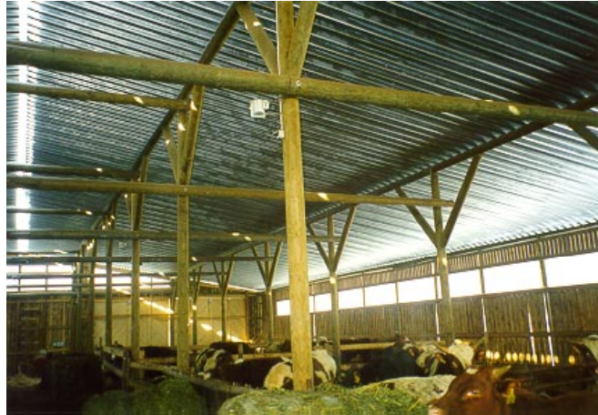
Figure 5.48 An uninsulated cow-shed in Viitasaari, 25 x 40 m.
