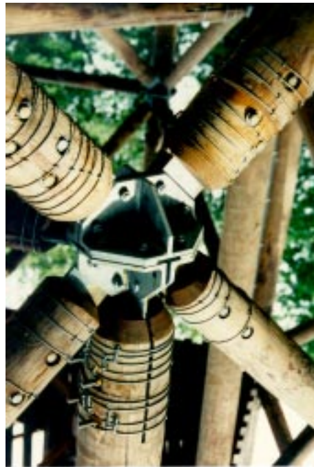
Figure 5.41. Pole joint in the Apeldoorn tower.
