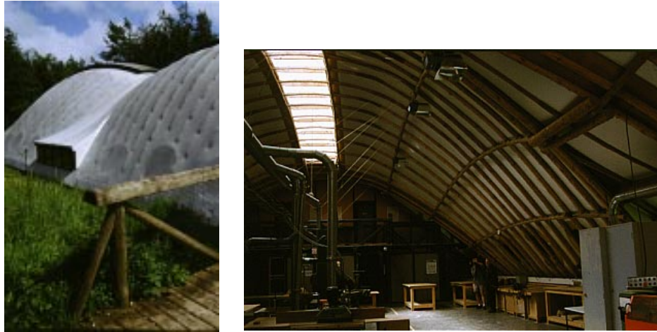
Figure 5.45. External and internal views of the workshop building at Hooke Park.
