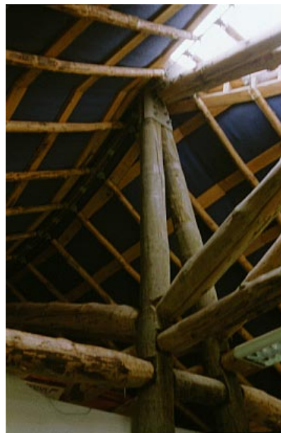
Figure 5.42. Interior A frame and rafters in prototype house at Hooke Park.
