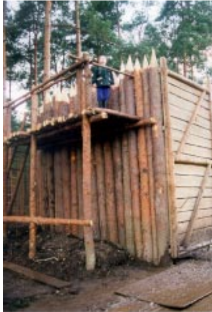
Figure 5.5. Round-pole ramparts and wall in f film set for a Roman fort.
