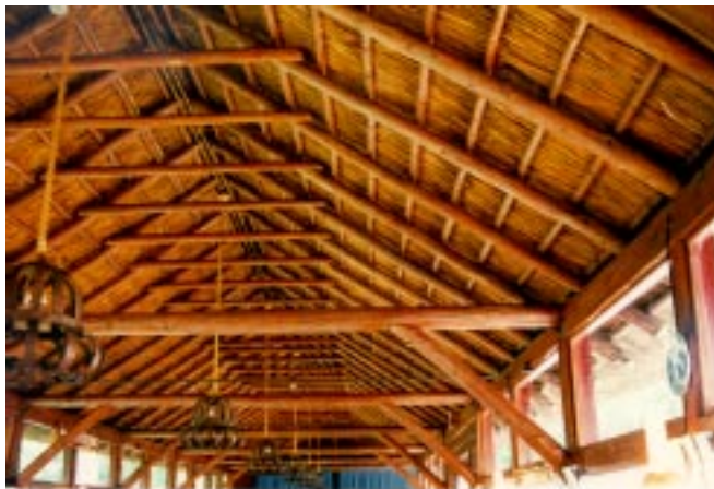
Figure 5.8. Tea-room at Apeldoorn. Both Figures 5.7 and 5.8 show adaptations of designs from traditional buildings in Dutch colonies in the Far East.
