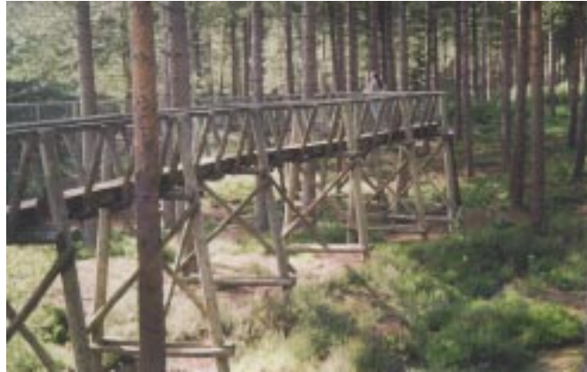
Figure 5.16. Bridge forming part of a tree top trail at West Moors.
