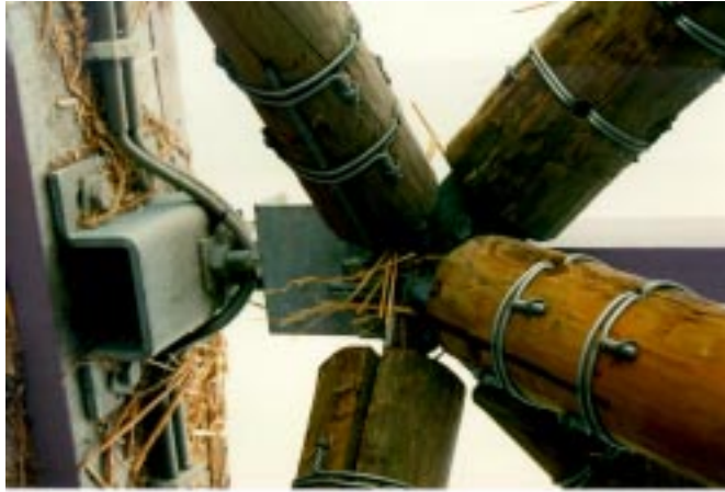
Figure 5.29. Huyber's space frame joint detail.
