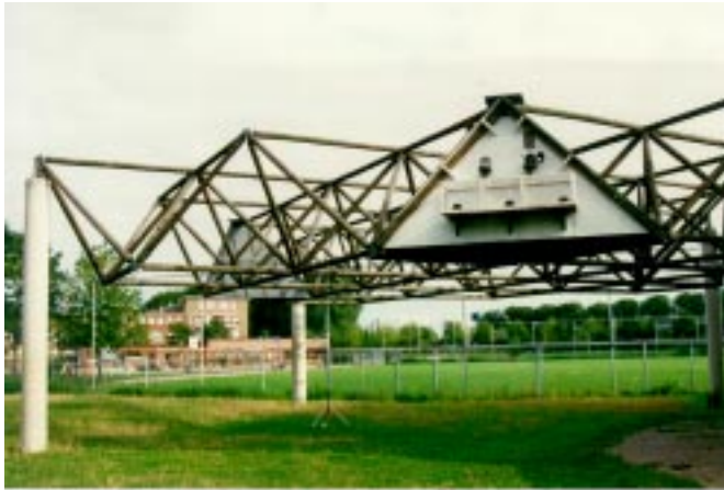
Figure 5.28. External space frame with bird houses in a children's zoo in Holland.
