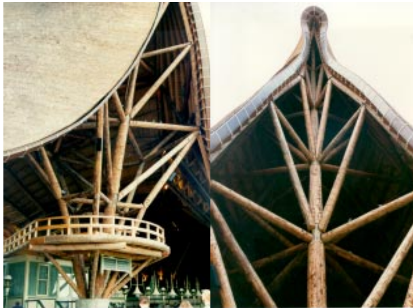
Figure 5.37. Two views of the Efteling structure in Holland showing the use of roundwood with other materials.
