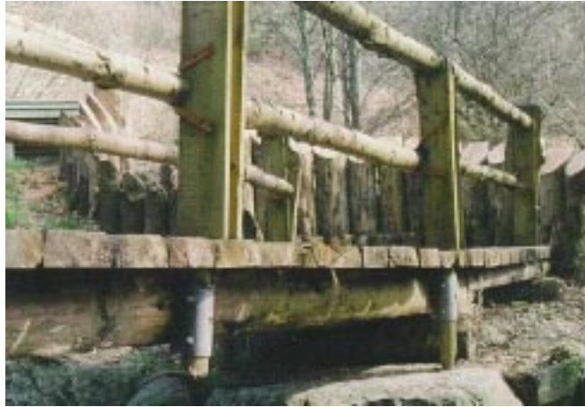
Figure 5.34. A simple footbridge at Castell Henllys in Wales using round-poles, main girders and hand rails.
