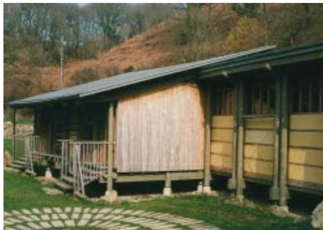
Figure 5.24. A visitor centre in Wales making good use of round-poles of different diameters.
