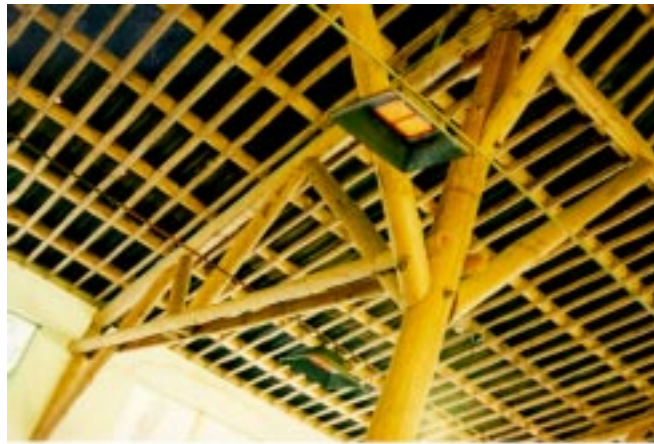
Figure 5.7. Restaurant roof in woodland park near Apeldoorn in Holland.
