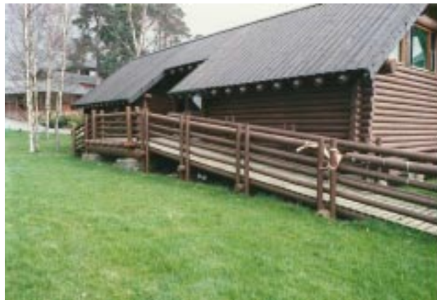
Figure 5.20. A large log house used as an exhibition centre in Wales, note also the use of round-poles in the entrance walkway.
