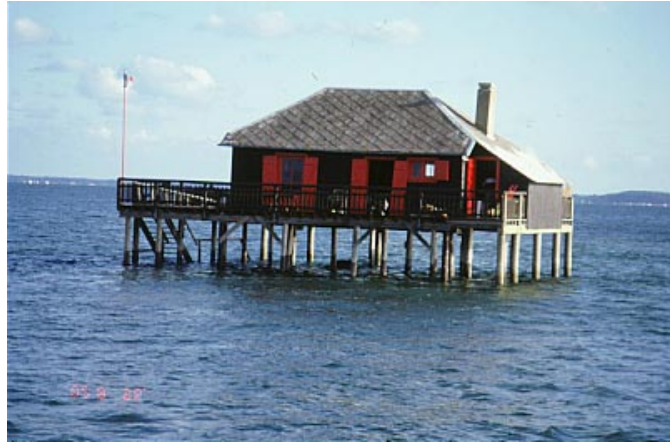
Figure 5.25. An extreme form of pole structure house built 6 m above ground level in France such that the floor is then above sea level.
