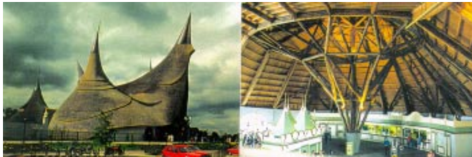
Figure 5.2. Two views of the Efteling building at Kaatsheuvel in Holland.
