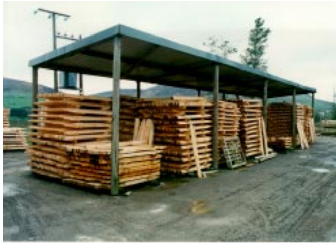
Figure 5.23. A very simple open barn round-pole structures used for drying fence posts in Wales.
