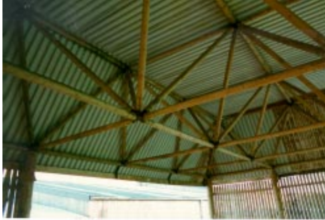
Figure 5.27. Space frame roof in barn in England.
