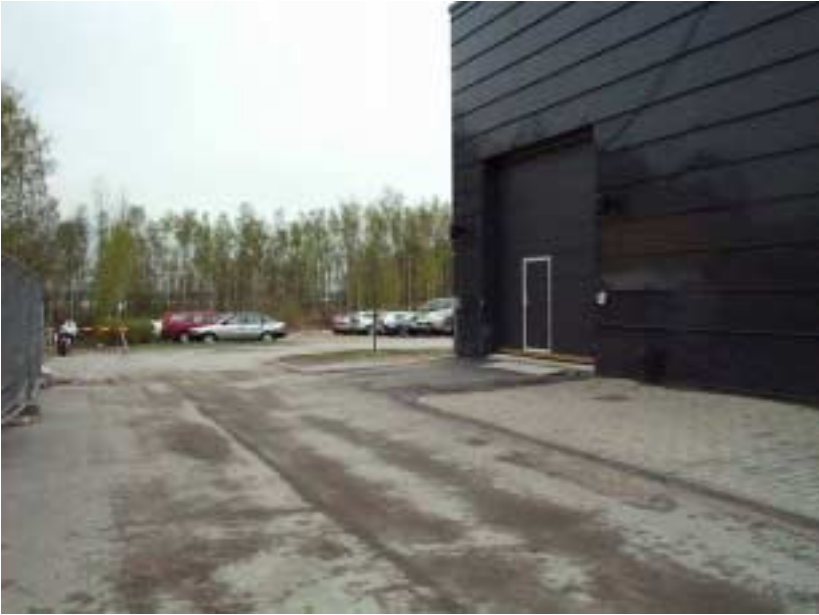
Figure 42. Test site for Workpartner.
