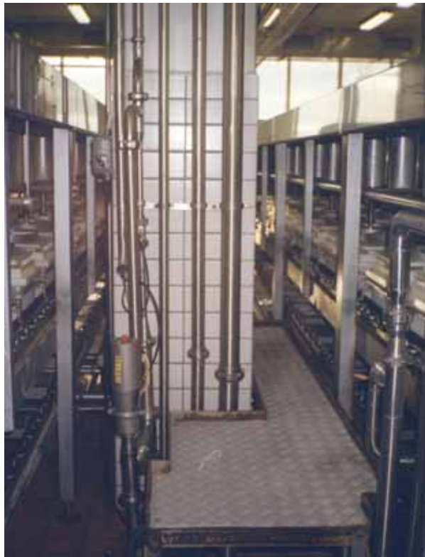
Figure 4.8. Processing area in Plant C.
