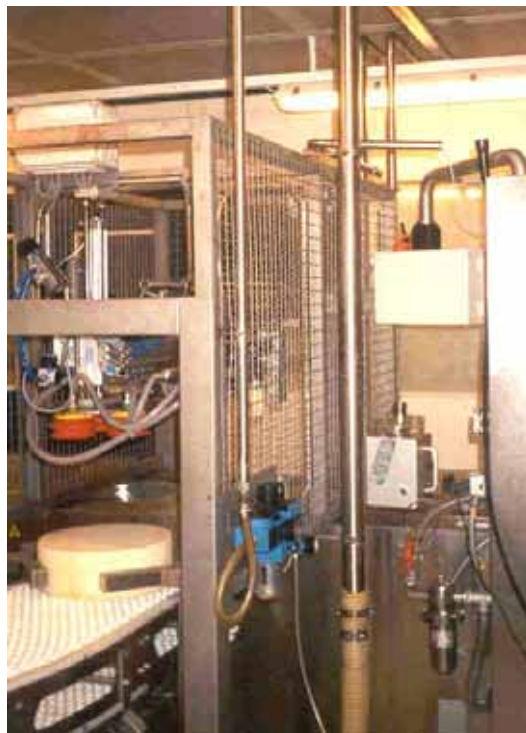
Figure 4.4. Packaging area in Plant A.
