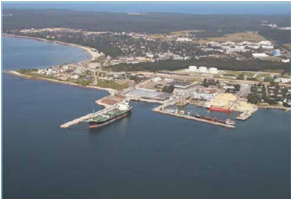
Figure 37. Miiduranna harbour area (Port of Miiduranna, 2004).
