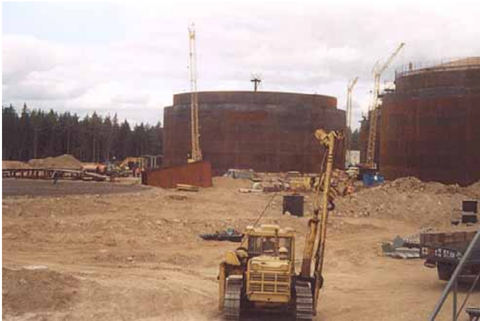
Figure 28. Construction of Vysotsk oil terminal, September 2003.
