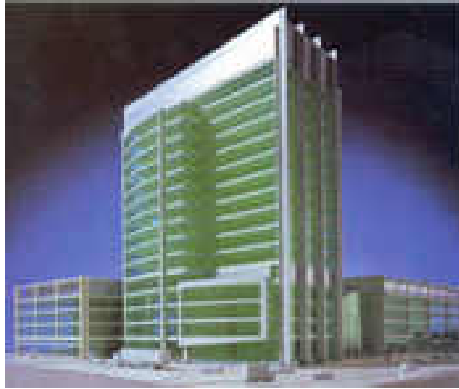
Figure 6.10. EGA Wing, Main Building Tower and Podium from the North (UCLH, 2002).
