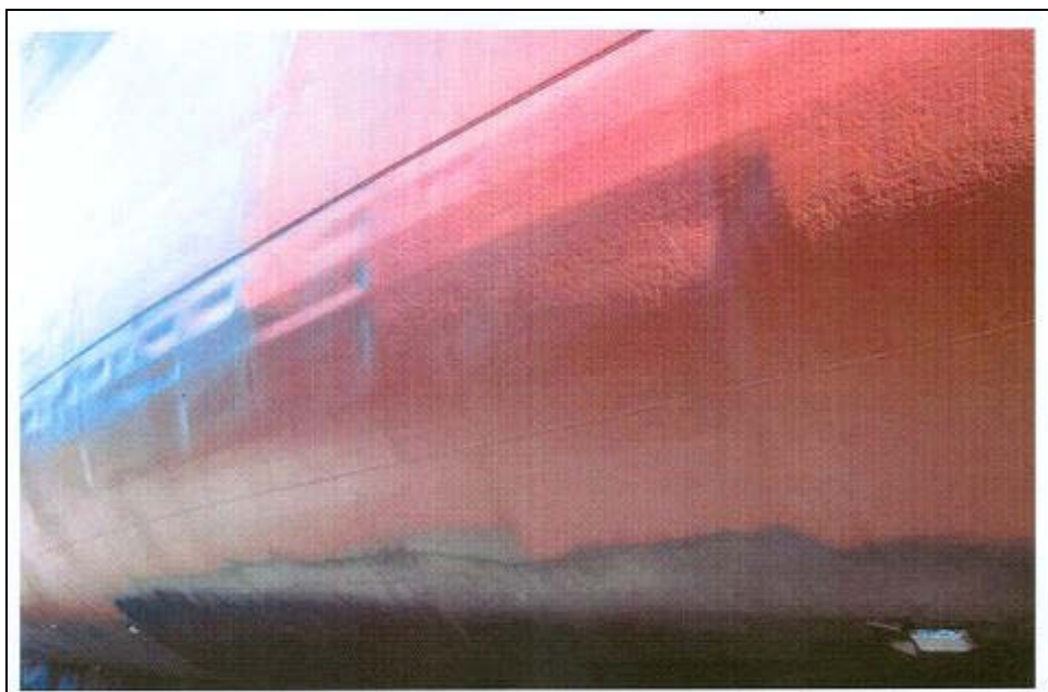
Figure 15. Observed damage to a chemical tanker of 22,700 DWT, ice class IA in winter 2003. The damage type is up to 25 mm deep dents on mid ship below the ice belt. Plate thickness of the ship was 14 mm, frame spacing 800 mm, frame span 2.4 m (Hänninen & Jalonen, 2003).
