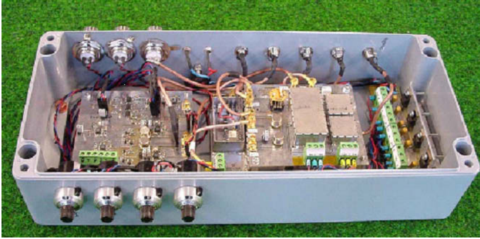
Figure 41. Photograph of the DC voltage reference.
