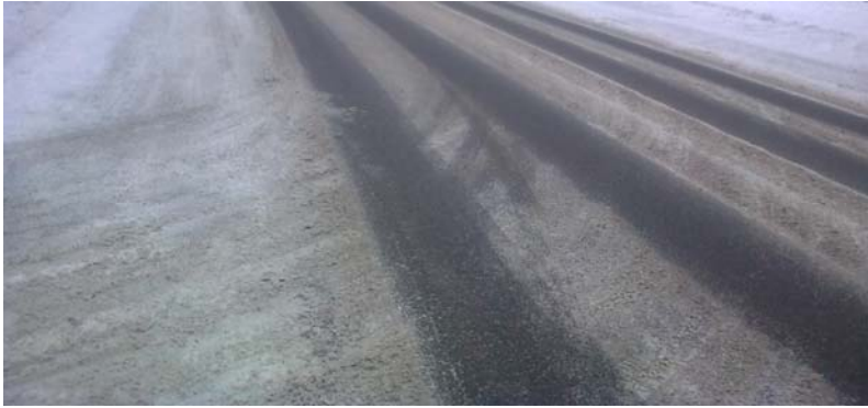
Figure 72. Varying surface type and friction potential cause difficulties in modelling the road – snowy road with clear asphalt tracks.
