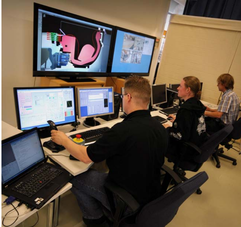
Figure 7.3. Upgraded control room.
