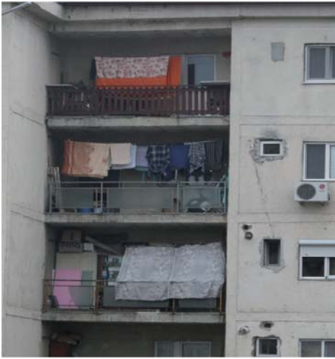
Figure 2. Improper use of balcony space as storage areas
