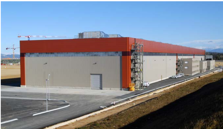
Figure A.3. Construction is now finished on the first building atop the ITER platform: the Poloidal Field Coils Winding Facility. Photo: F4E January 2012.
