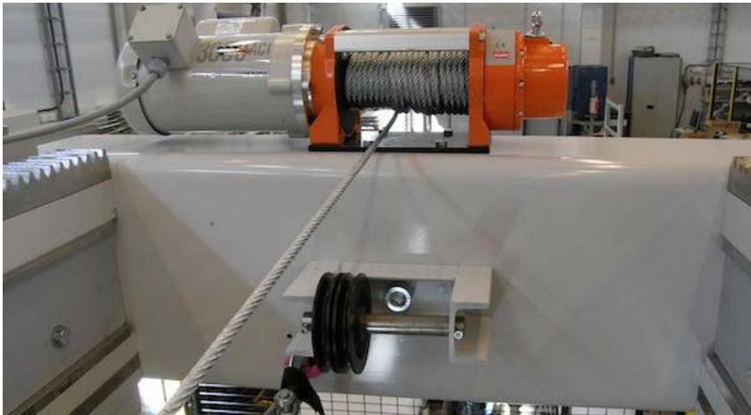
Figure 6.1. Rescue operation of CMM/SCEE + Divertor cassette using pulling device, which is installed to the end of the radial rails.
