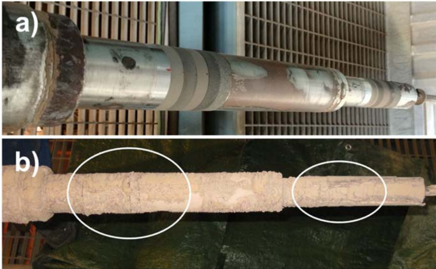
Figure 19 Probe a) before exposure and b) after 5900 h exposure in the biomass co-fired boiler. Left: specimens exposed at 550 °C. Right: specimens exposed at 750 °C.
