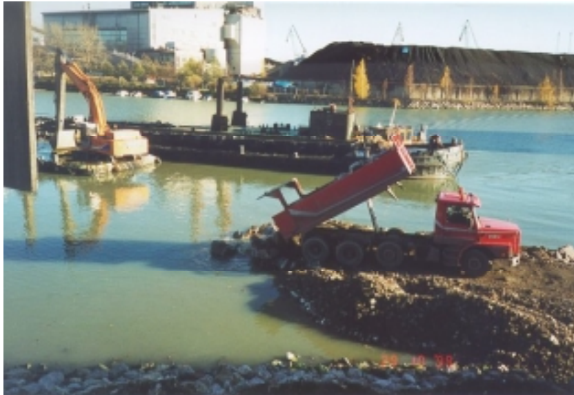
Figure 3. Dredging and building of the edge embankment in Sörnäinen, Helsinki.
