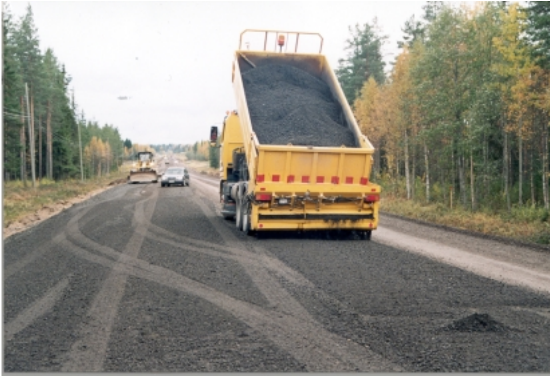
Figure 1. Pulverization in a bearing layer.
