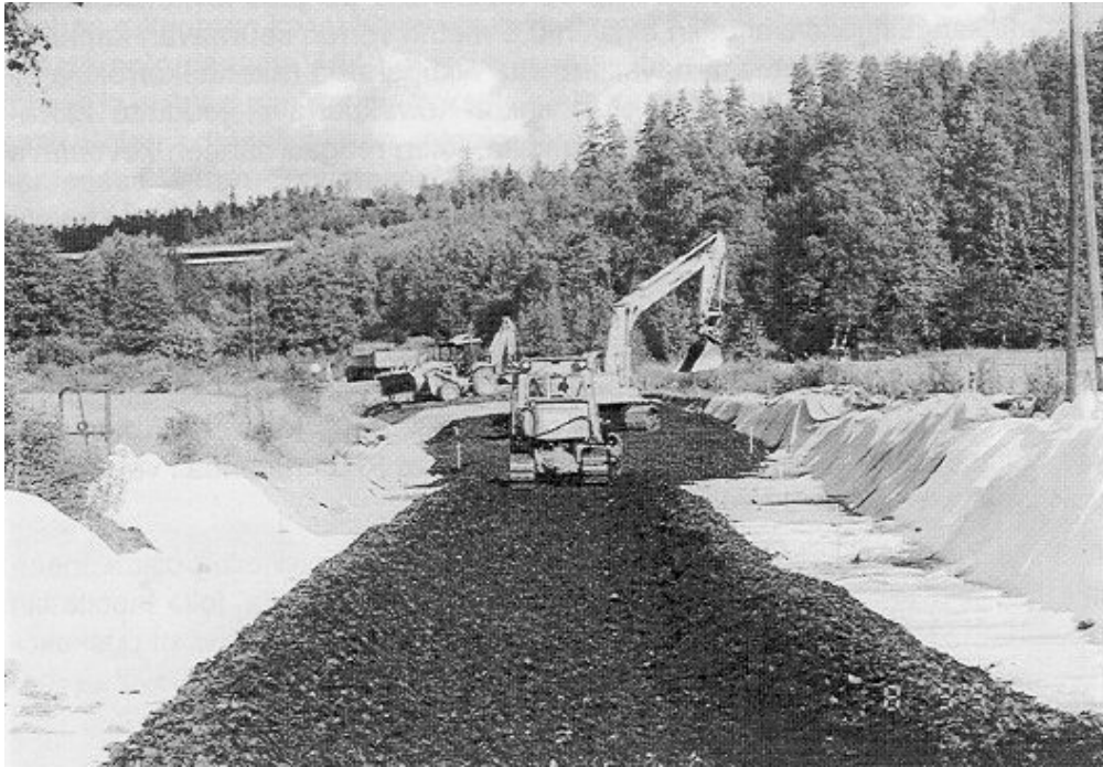
Figure 1. Constructing the pilot structure.
