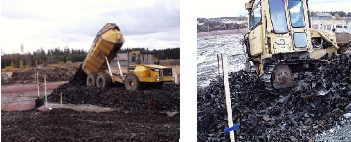
Figure 3. Construction of the RR1 tyre chip layer.
