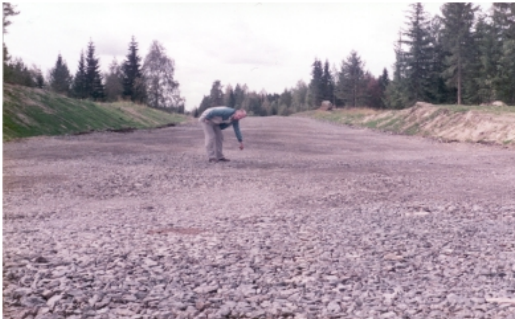
Figure 2. Air-cooled blastfurnace slag as a sub-base and bearing layer.
