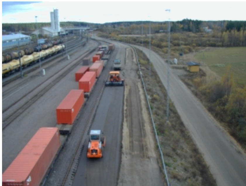
Figure 5. The finished Ekostab-product was used by the client as a pavement base material.
