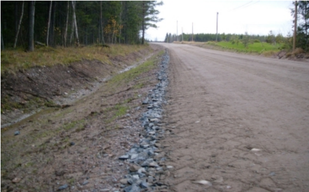
Figure 6. Dust binding on the wearing course of a clay-gravel road.
