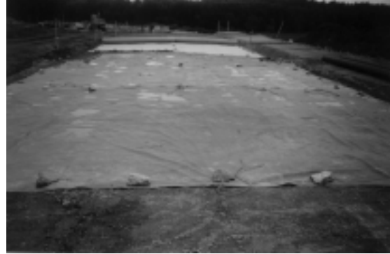
b) Clay mass covered using plastic.
