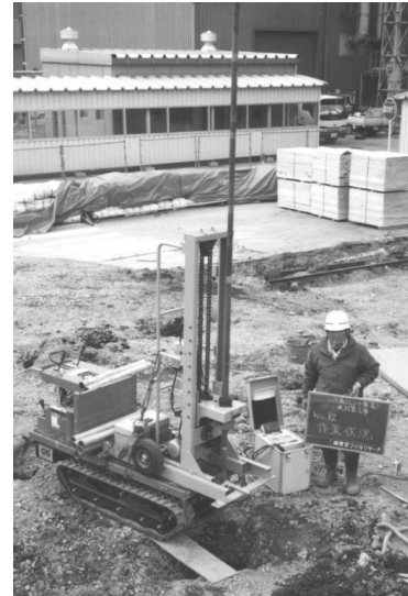
Photo 4. Shallow depth boring machine mounted on a mini caterpillar.
