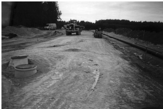
c) Constructing clay-road.
