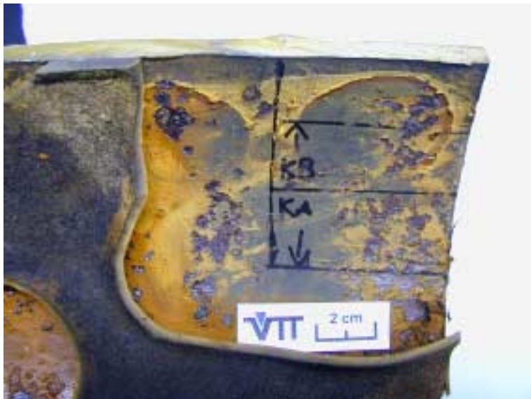
Figure 3. Surface of the steel under the large rubber blisters is not heavily corroded.
