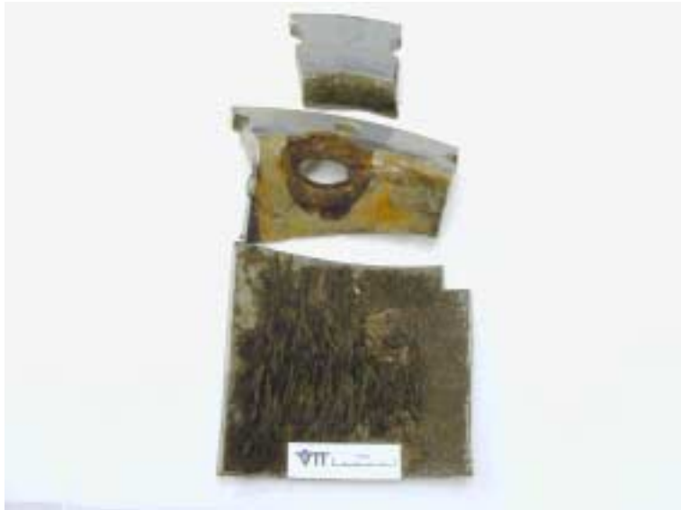
Figure 2. Painted seawater pipe having a breakthrough hole adjacent to the flange.
