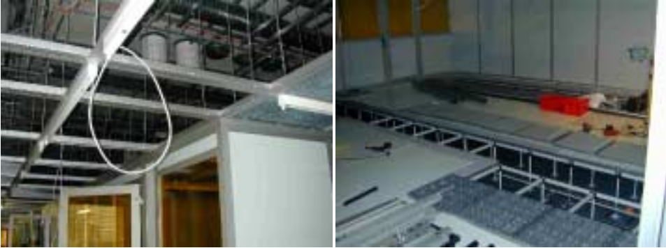
Figure 1. Clean room construction.
