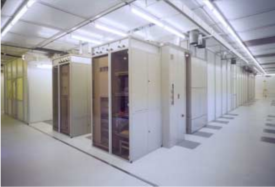
Figure 4. View of surrounding corridor showing diffusion furnaces.
