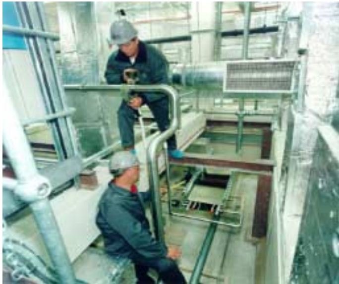
Figure 8. Remember access to the work during installation.
