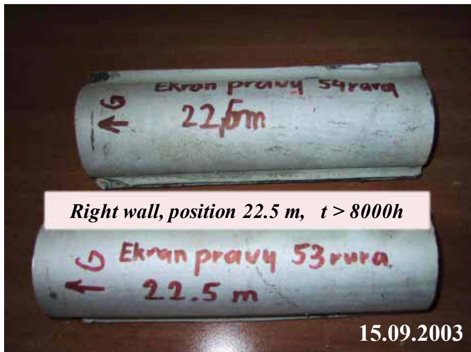
Figure 8. Photograph of the water wall tubes protected by HybridMD coating after 8000 h operation in "Siekierki" Power Plant.
