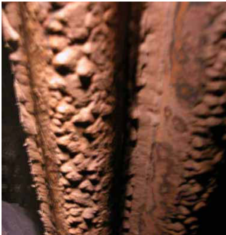
Figure 5. Roof tube surfaces after sand blast cleaning.
