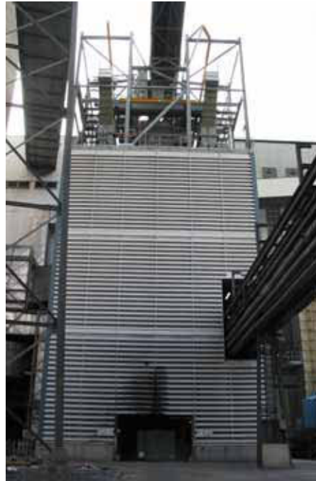
Figure 3. The Ruien gasifier building.
