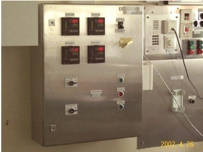
Figure 47.4. Zoned controls with temperature correction possibilities.
