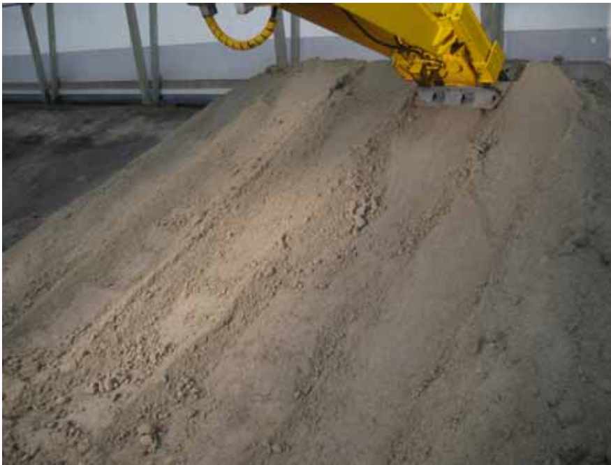
Figure 2. Compaction of the inclined layers. Photo: D. Adam.
