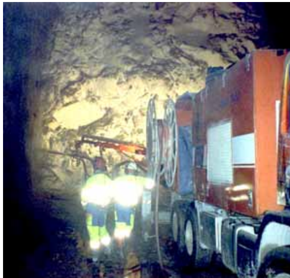
Figure 9. Shotcreting of the blasted tunnel end in October 2002.
