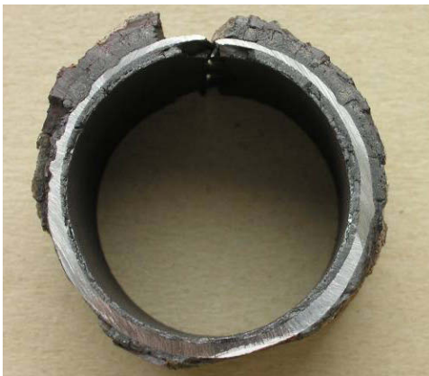
Figure 3. Double sided wall tube thickness losses are visible.
