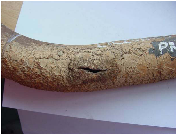
Figure 7. Place of failure.
