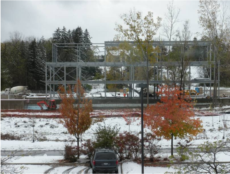
Figure 8. Erection of a 60,000 square feet office steel framed building.
