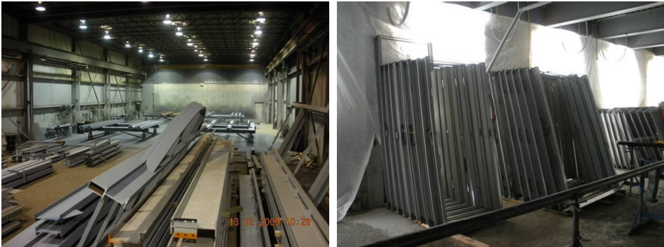
Figure 10. Tracking of prefabricated assemblies indoors, either at a fabricators warehouse or at a construction site, poses difficult challenges. Left picture shows structural steel assemblies at the fabricators warehouse awaiting shipment. The picture on the right shows the doors and windows assemblies at a construction project.
