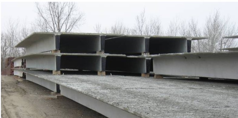
Figure 9. Precast concrete elements stacked in layers.
