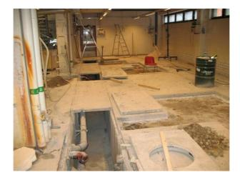
Figure 1. Replacement of floors and drains.
