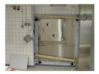
Figure 2. The 'wall-integrated' freeze dryer during installation.
