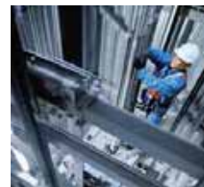
Tytyri elevator testing facilities
