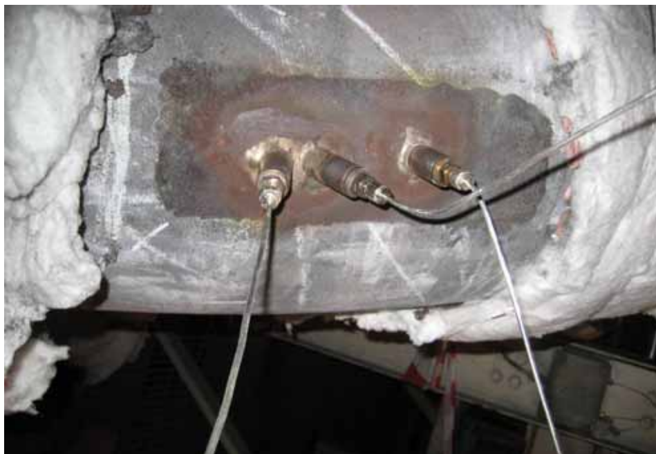
Figure 1. High temperature probe installation at Ratcliffe in 2007.
