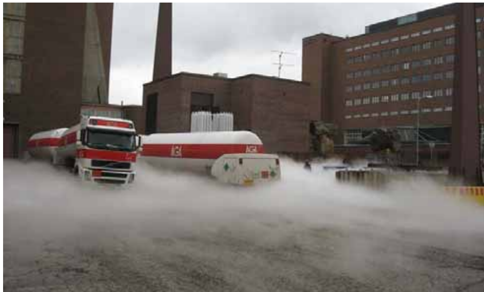
Figure 4. Nitrogen injection at the Salmisaari power station.
